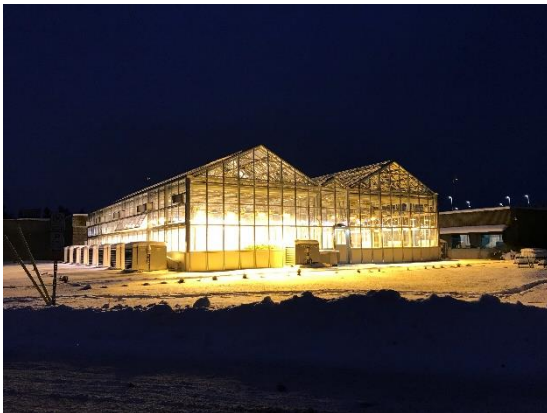
High intensity lighting system
