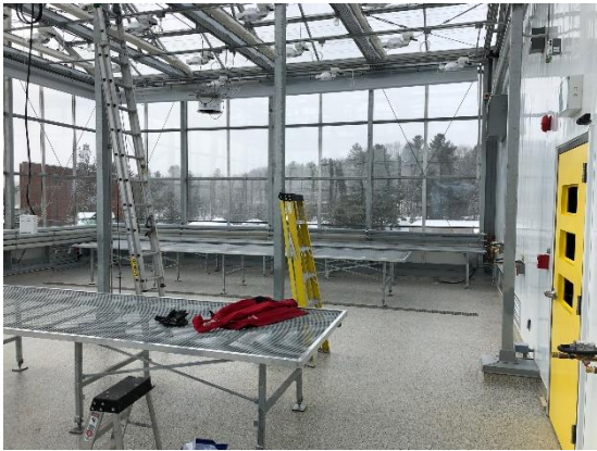
Inside of the greenhouse space, at end of construction phase
