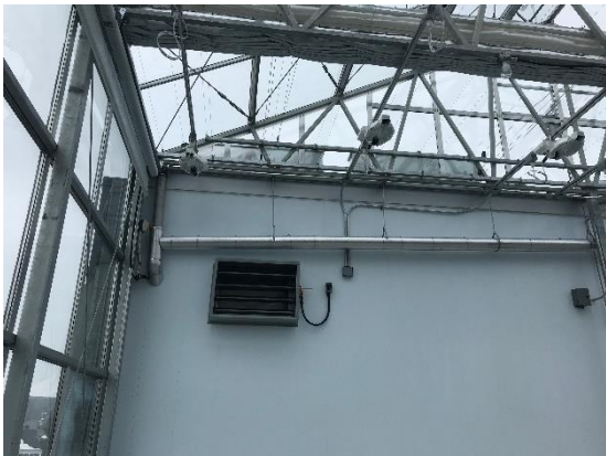
Rainwater harvesting system
