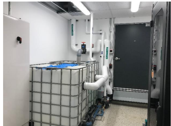
Rain water storage tanks
